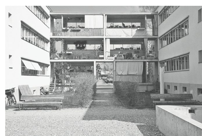
Vogelbach-Housing Development, Michael Alder
